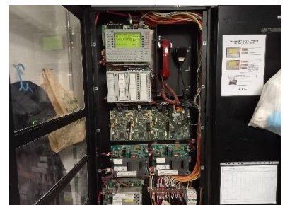
Fire Fighter Telephone System
