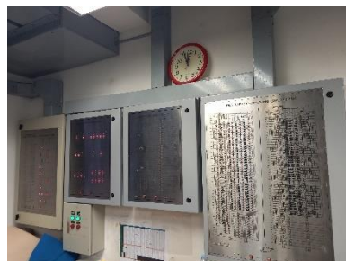
Graphic Annunciator Fire Alarm System
